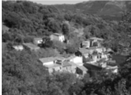
Buildings in ruins
