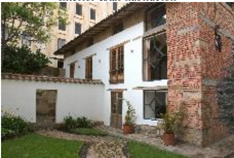
Fachada patio interior
