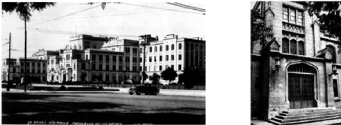
Fig. 8. General view of the new building of the Medicine School (1931), São Paulo, and detail of its main entrance. In Três Escolas de Medicina de São Paulo . São Paulo: Santa Joana Hospital e Maternidade, p. 15 and p. 24.
