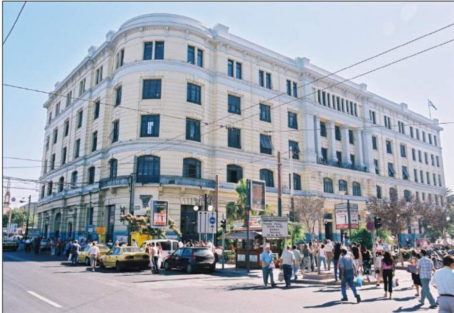
Fig. 4. Greek Electric Railways (EHS) Mansion in Piraeus. External view (1926)
