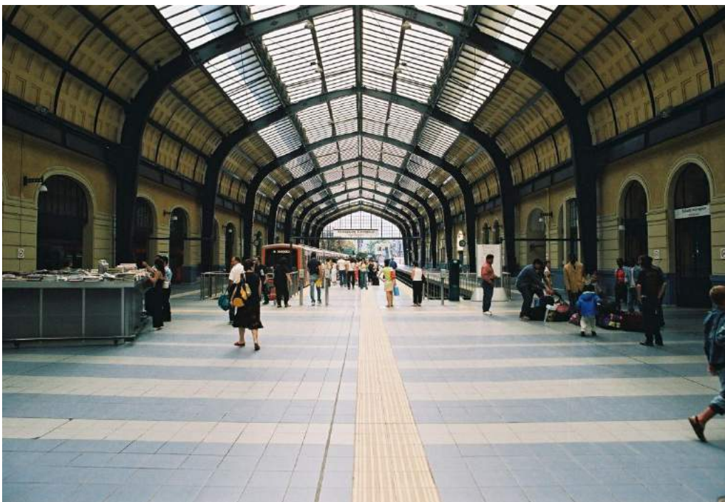
Fig. 6. Interior view of the Piraeus Terminal Electric Railways Station (ISAP) today (2016)
