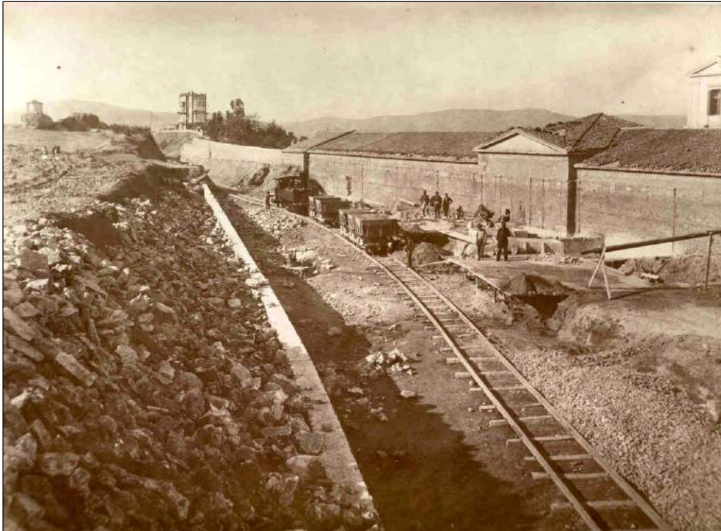
Fig.1. Athens-Piraeus Steam Railway Line (SAP) under construction in Thissio area. (1869)
