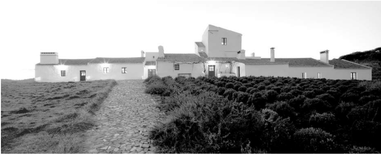
House, Vila Boim
