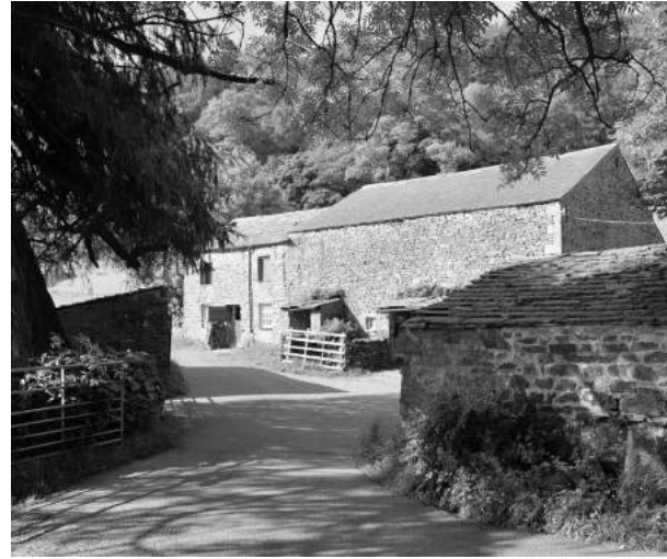
Farm buildings at Brackensgill, Dent. (a former Long House). Henk Strik
