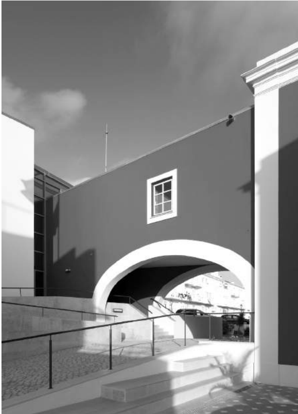
Assisted Residence, Sines
