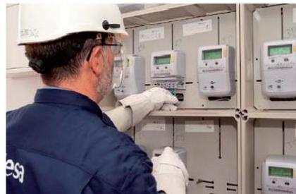
Figure 2. Placement of smart meters by an Endesa operator in the Smartcity in the framework of Málaga Project. Source: [3]
