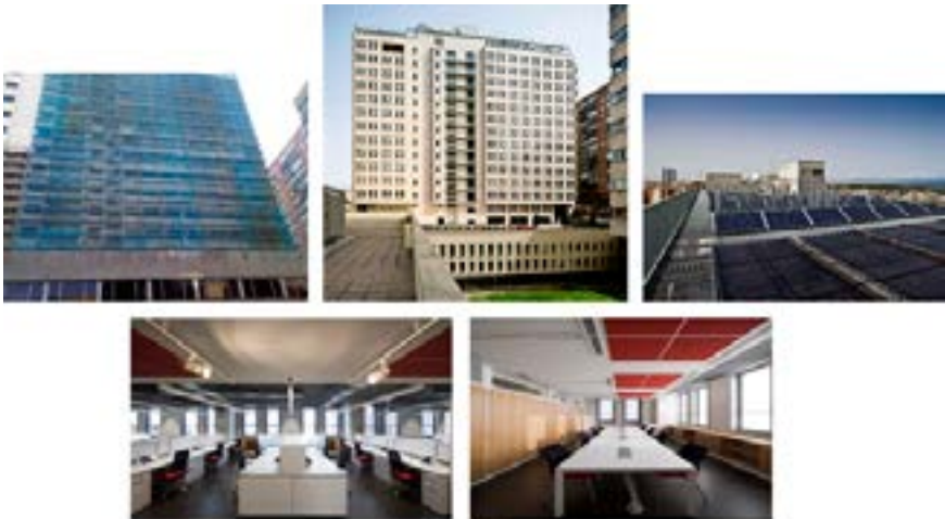
Figure 5- Major refurbishment of the ISDEFE S.A building. (Source: Presentation "ISDEFE Headquarters. From obsolete to efficient and smart building. A Defence example", CF SEDSS Phase 1, ISDEFE, Spanish Ministry of Defence, Thessalonica 2017).
