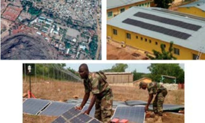
Figure 4- Aerial view of the Koulikoro Camp; Building 55 at the Koulikoro Camp; Forces deployed at the Koulikoro Camp installing flexible photovoltaic panels.
