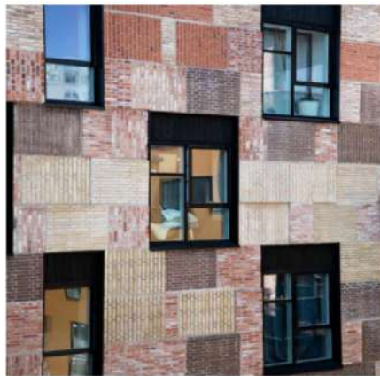
Figure 2. Patchwork facade of the Resource Rows residential complex (built with masonry panels obtained from the deconstruction of the Carlsberg Brewery, Copenhagen, Denmark).
