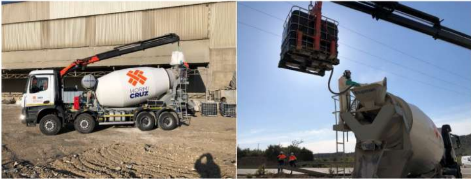
Figure 6. Introduction of the materials inside the concrete mixer.
