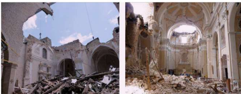
Figure 5. Typical seismic collapses of masonry and timber covers and supporting elements by the L'Aquila, Italy EQ in 2009, Mw= 6.3,
