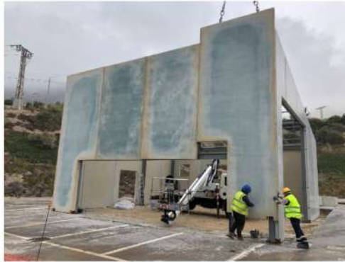
Figure 14. Placement of the fourth and last plate of the facade.
