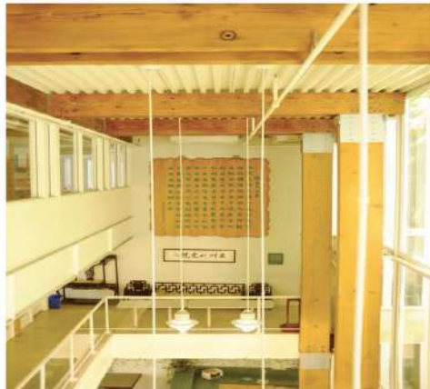
Figure 6. Interior of the C.K. Choi Building showing the use of wood components from the former Armoury for structural purposes Source: Ross, (2020).
