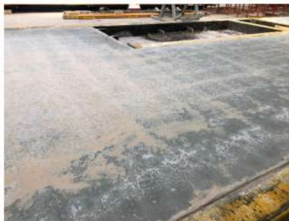
Figure 10. Detail of the surface of the plates 24 hours after pouring.
