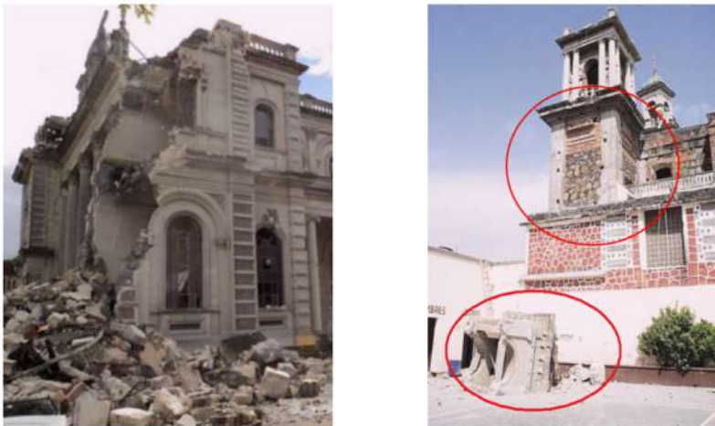
Figure 6. typical seismic collapses of masonry bell-towers: a) damages by the 2011 Christchurch, New Zealand EQ Mw= 6.3, Source: Lester et al. (2012) and b) damages by the 2003 Colima, Mexico EQ Mw= 7.3, Source: Preciado (2011).
