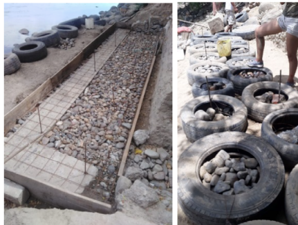
Figure 8. Wall construction start-up process. Source: Eduardo PeñalozaKairuz (2019)
