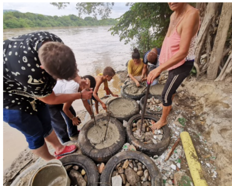
Figure 9. Wall construction process Source: Eduardo PeñalozaKairuz (2019)
