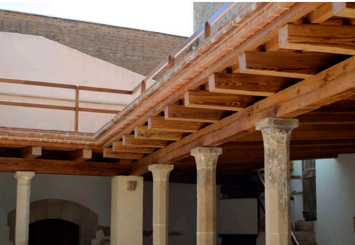
Restored wooden members of the Cats' Cloister
