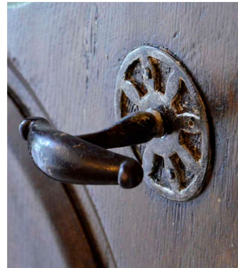
Window and door fittings in the Palace of Trénor
