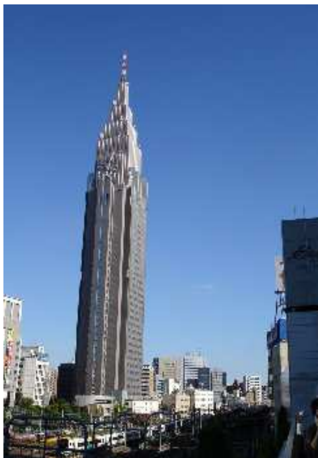
Figura 6.19: NTT DoCoMo Yoyogi Tower, Tokyo, 1997-2000, NTT Power and Building Facilities. Fotografía: Lye Gunnstein.
