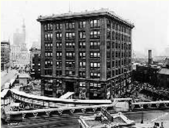
1930 Indiana Bell Telephone building on the move
