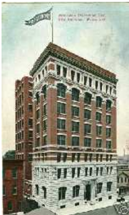
Figura 3.38: Wisconsin Telephone Co. , Milwaukee, Alexander Eschweiler 80 , 1905-1907.
