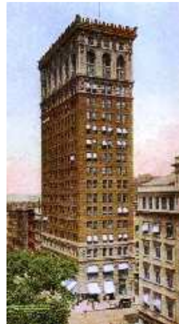
Figura 3.35: Chambers Building , 1889-1890, Cass Gilbert.
